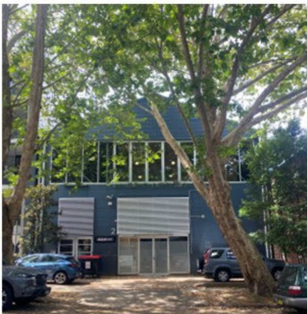
View looking east on Hunter Street along frontage of site.
