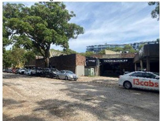
View looking south on Young Street along frontage of site.
