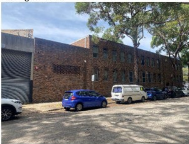
View looking east on Hunter Street along frontage of site.
